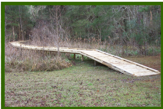
A new boardwalk is completed over a bog garden.
